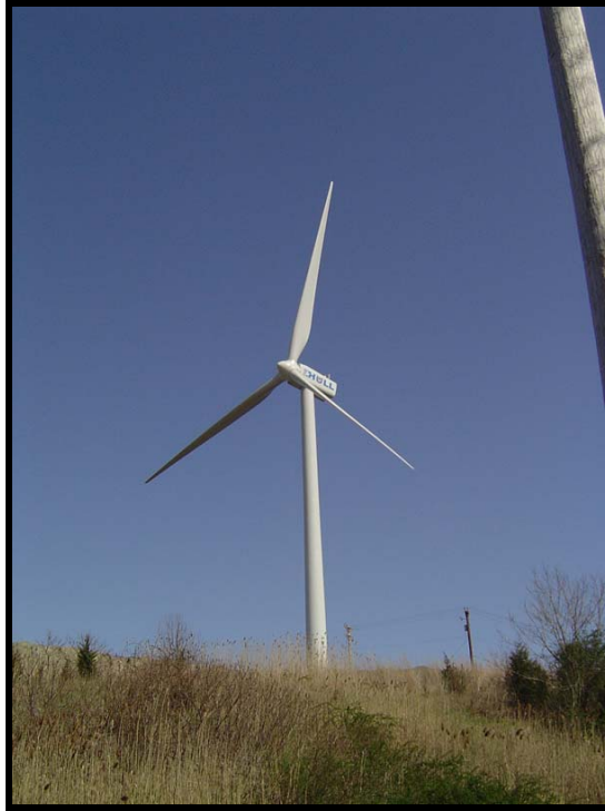
Figure 1.1 – Vestas Turbine at Hull, MA project
