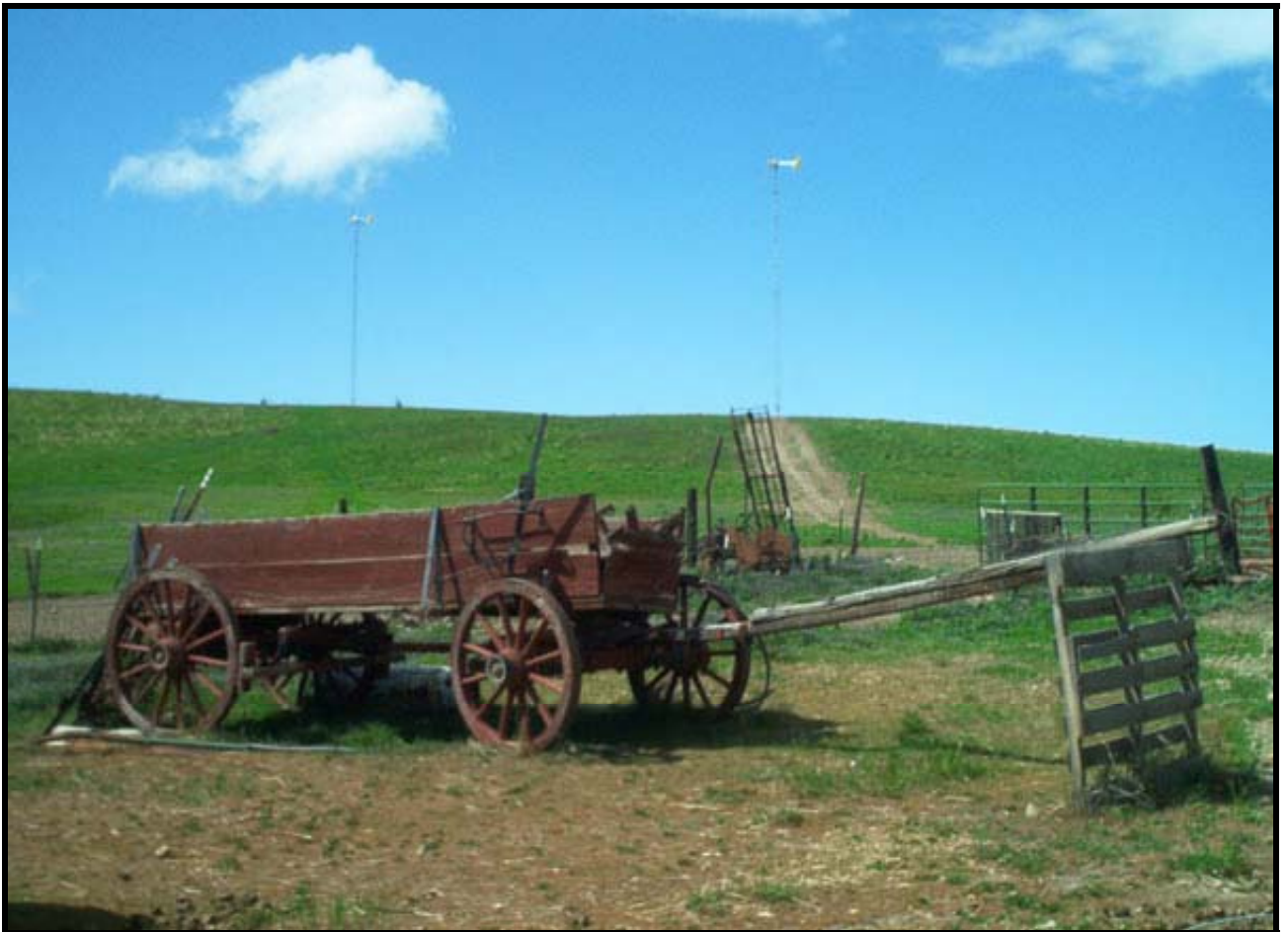
Figure 4.1 – Bergey Excel Turbines on the Kingsbury Wind Farm
