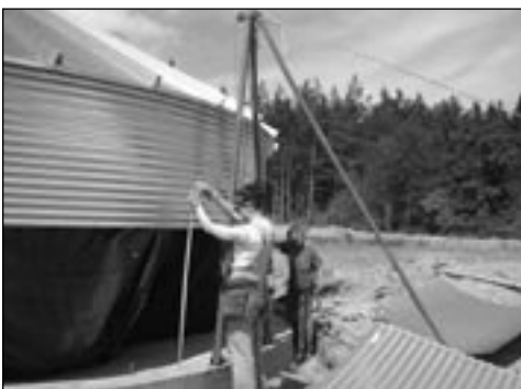
Interns installing the rainwater tank
