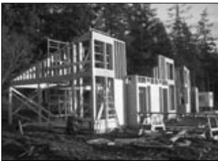
Framing the office and rentals
