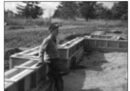
Contractor Pamela Pauly with foundation
